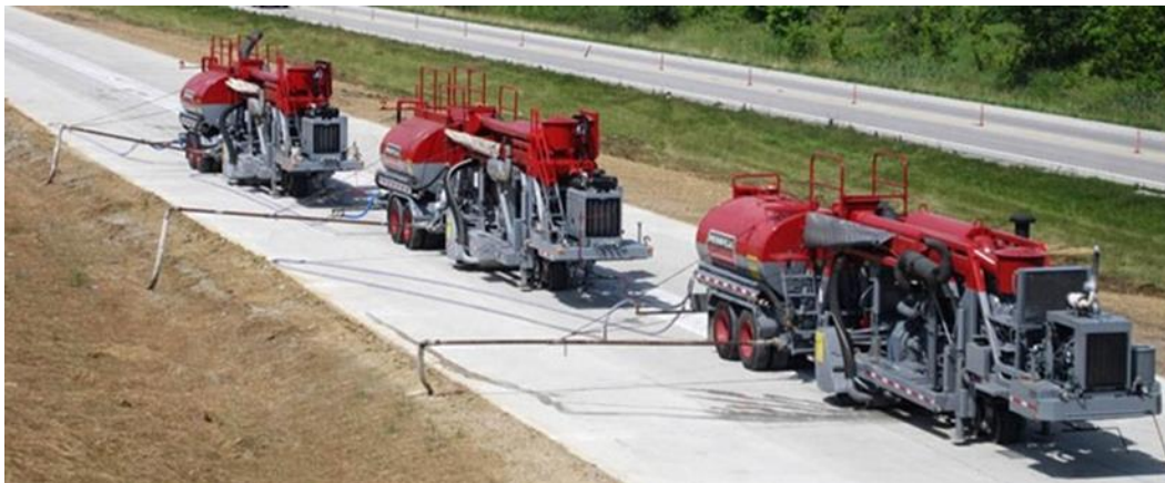
Figure 7: Side Slope Slurry Spreading (Penhall 2014)
